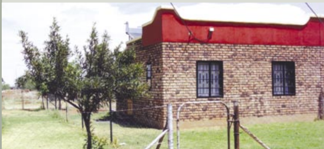
Trees, shrubs and grass have been planted around the development to provide greenery
