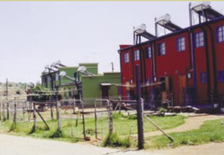
Double gates allow cars to access the parking space on each plot
