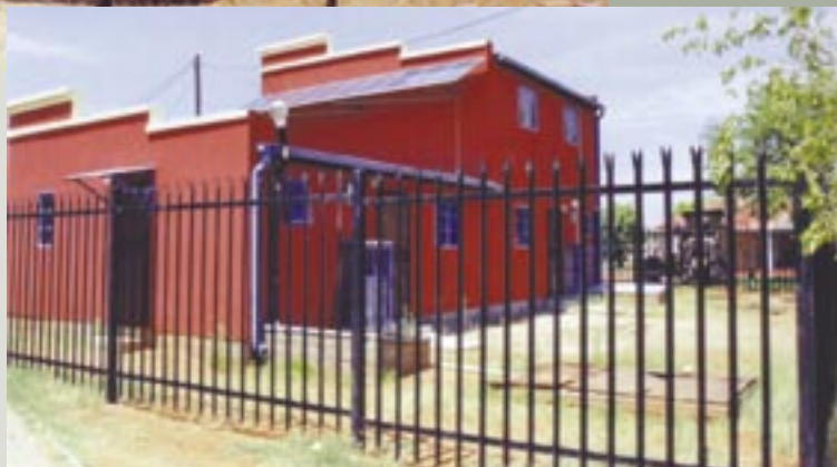
Palisade fencing secures the perimeter of the development
