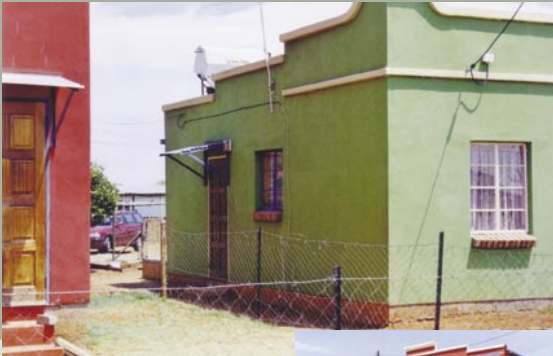
Windows on the front and sides of units encourage the use of natural lighting within
