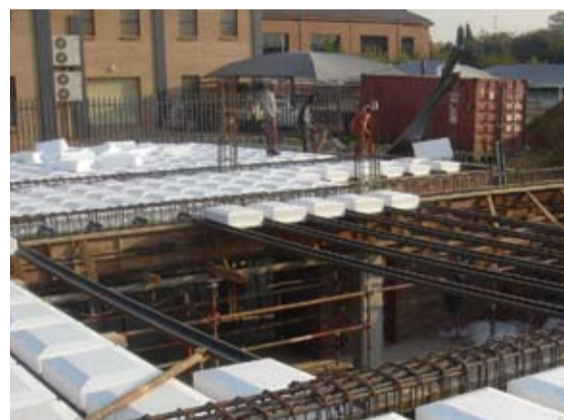
Innovative construction techniques are beginning to penetrate the local building industry.
